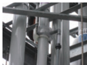
Double joints in piping Installation of double joints in piping to enable checking for leakage of fluids
