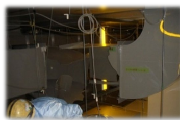
(c) Damage to Local Exhaust Duct
