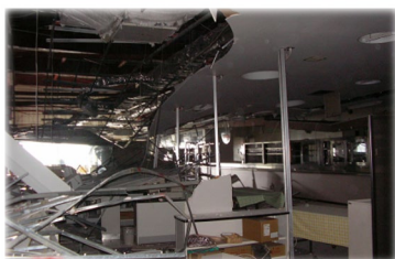
(a) Ceiling Collapse
