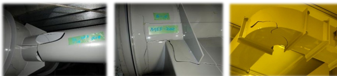
Figure 6. Duct Damage (Cracks, Breaks)
